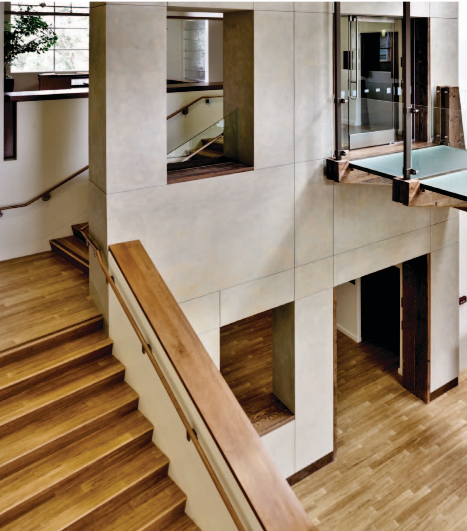
For the Moore Foundation headquarters in Palo Alto, CA, Mission Bell teamed with Blach Construction and HPS Architects using AutoDesk BIM (Building Information Modeling). Recycled and reclaimed materials were incorporated in this LEED Gold certified project, with a unique 'flying beam' design, glass bridge, and undulating recycled timber beams ©Marco Zecchin/Image Center.
